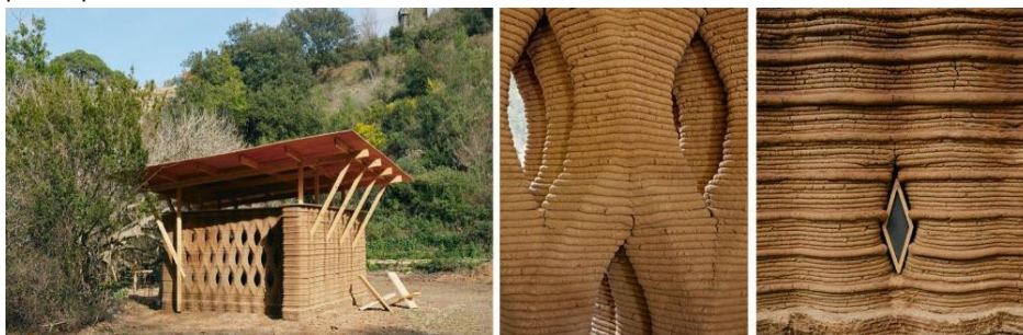
Figure 6. TOVA Prototype (left). Opening detail (center). Ventilation shaft (right), IAAC 3DPA 2021-2022. ©Gregori Civera
